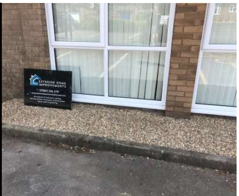
Improvements to the front of Richmond Surgery
